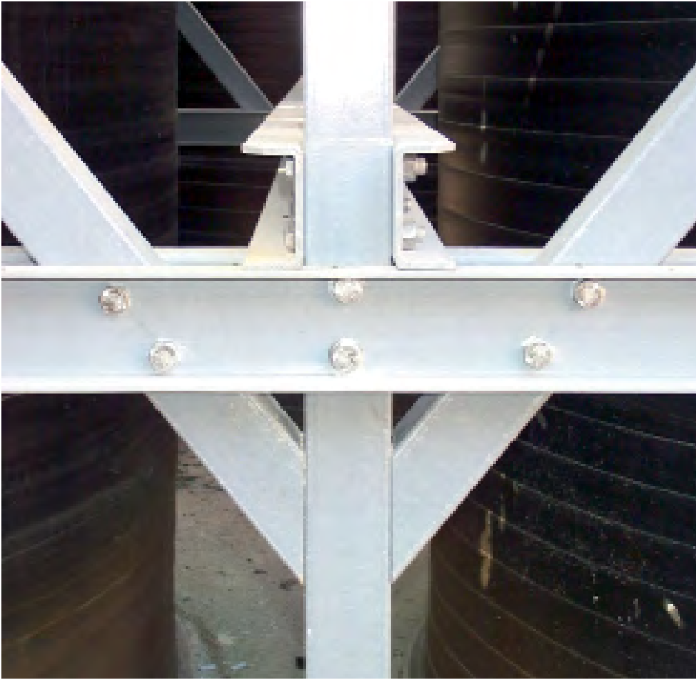
Top: Detail of a possible GRP structure
