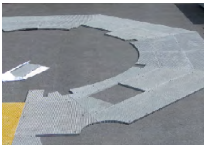
Bottom right: Quality control of GRP grating
